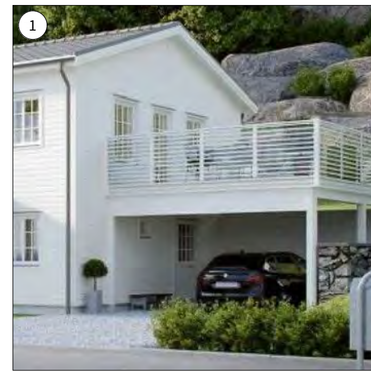
Future Deck for Garage Apartment + Shaded Carport
