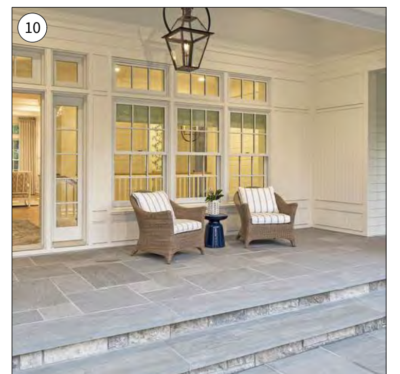
Stone Flooring on Porch and Extended Stairs
